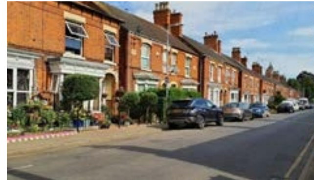
Cohesive building line along Tawney and Thorold Streets
