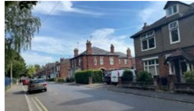
Linear static views along Thorold Street, channelled by the buildings, box hedging, kerblines and park railings.
