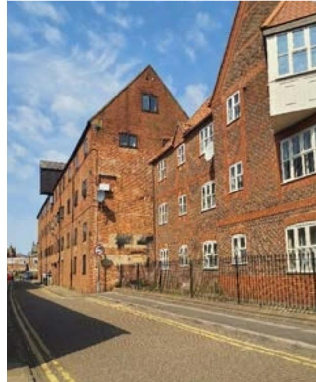
Setted carriageway of Spain Lane
