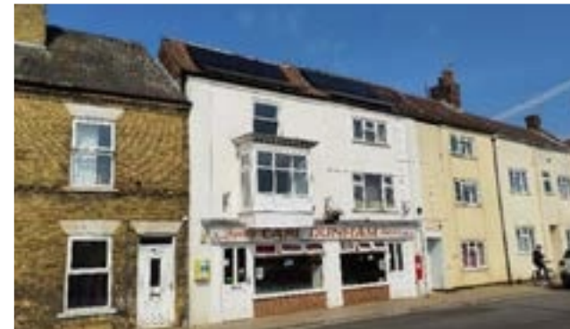
No. 16 London Road, Carl Dunham Butchers shopfront
