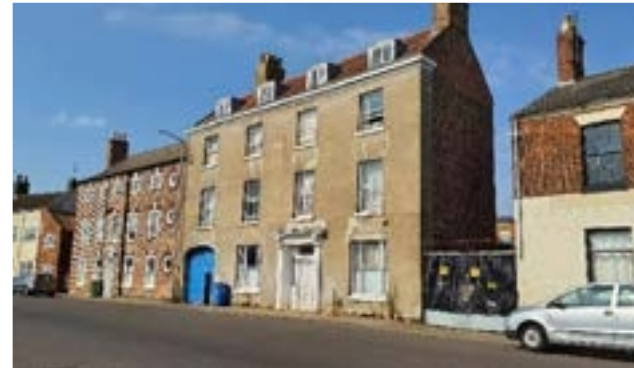
Urban grain along London Road in differing styles, reflecting the development, expansion and alteration of buildings in this area
