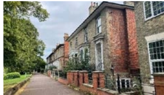
19th century houses fronting the river and with raised basements to allow views across the river
