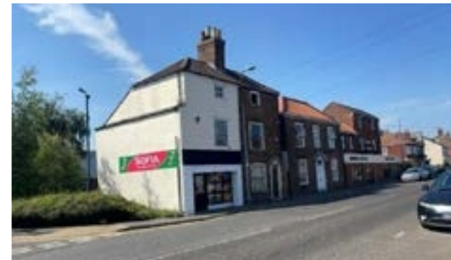
Mismatch of building styles and modern amendments fronting Horncastle Road
