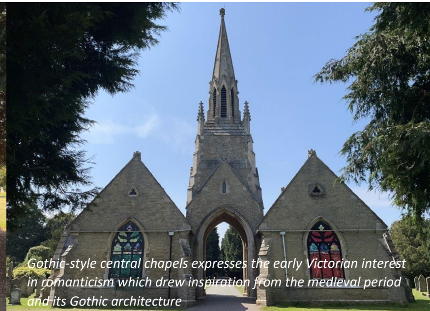
Carrigeway leading away from the chapel
